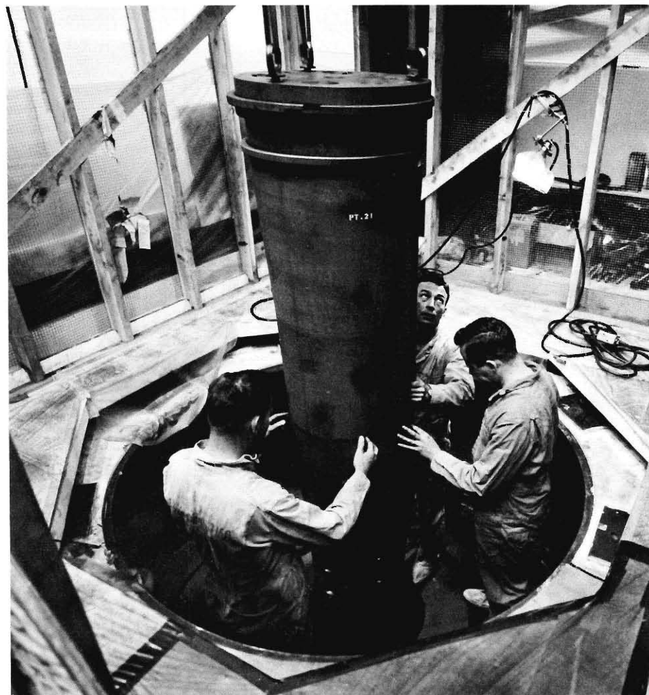
The UHTREX reactor core being lowered into its containment vessel.
