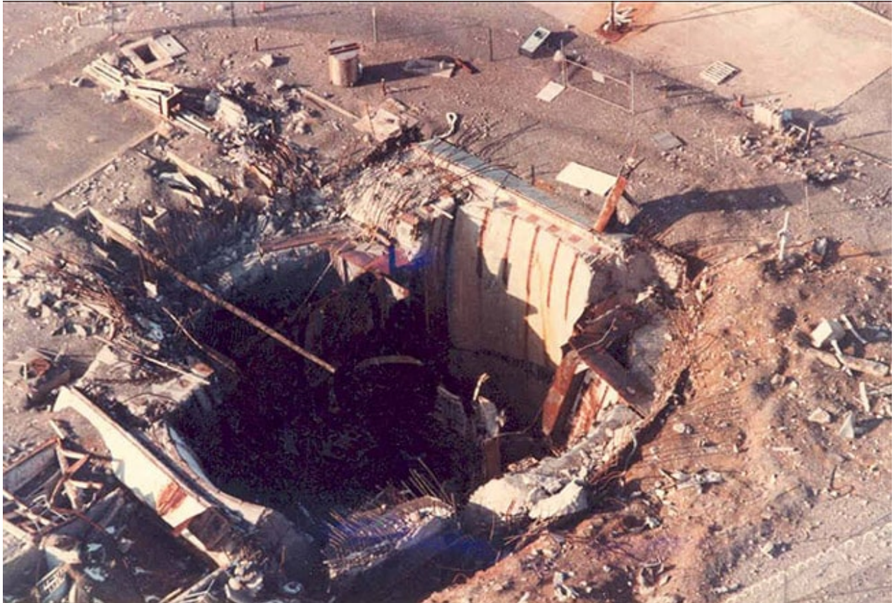
Aerial view showing damage to the Titan II Missile silo in Damascus, Arkansas, after the 1980 explosion. Image courtesy of airman Greg Devlin/ Encyclopedia of Arkansas
