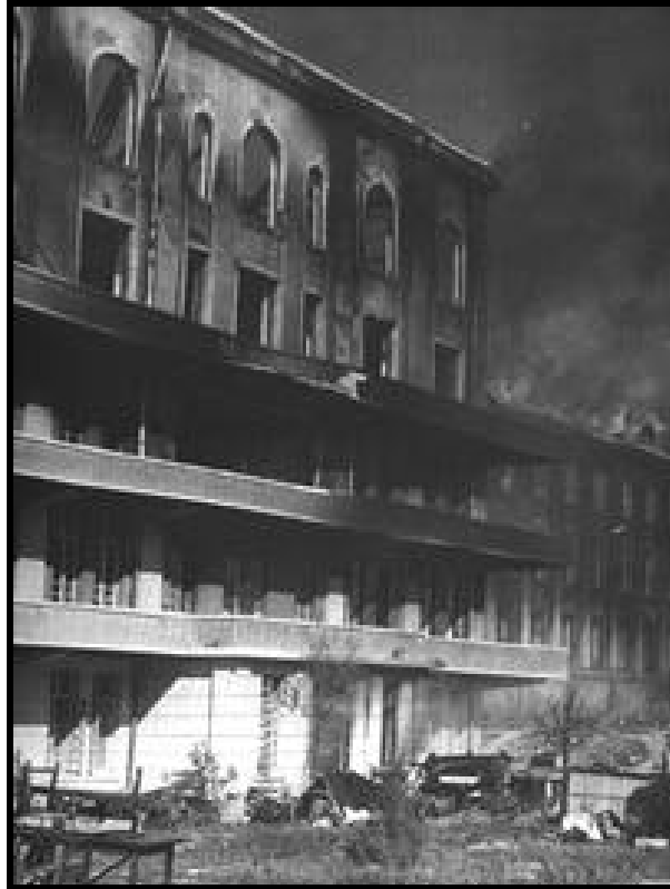
Figure 3.7: War-damaged Kim Il Sung University in 1953 [From: KCNA 96]
