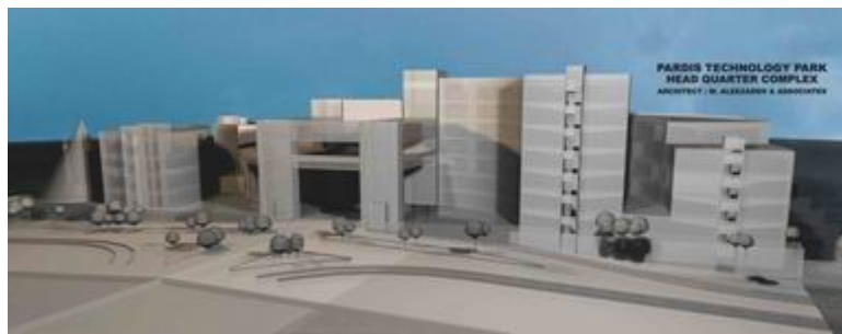
Figure 4. Pardis Technology Park Headquarters Complex [PTP 02]
