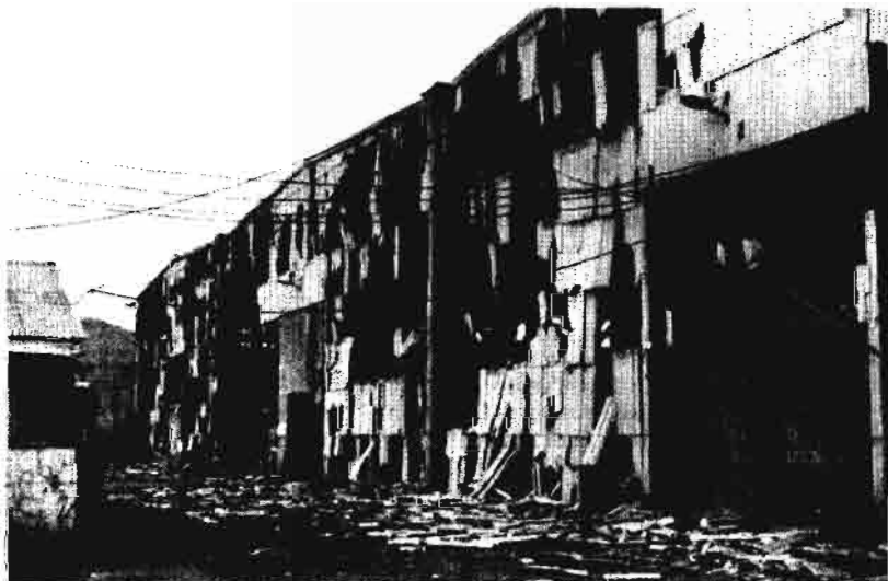
The ARDF aircraft hangar adjacent to the Bendix and Harris Corporation huts. Concussion caused most of the damage.
