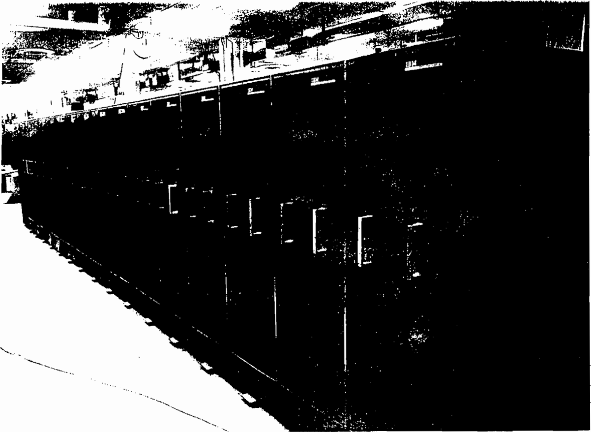
Figure 25 -- HARVEST -- The 16 Frames of the Central Processing Unit
