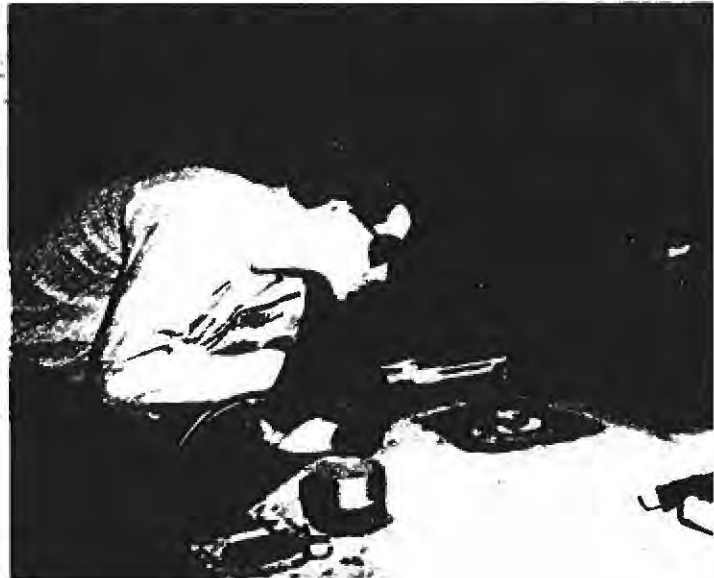
Danish construction worker cuts a filler pipe hole in the top of an R-4360 engine container.
