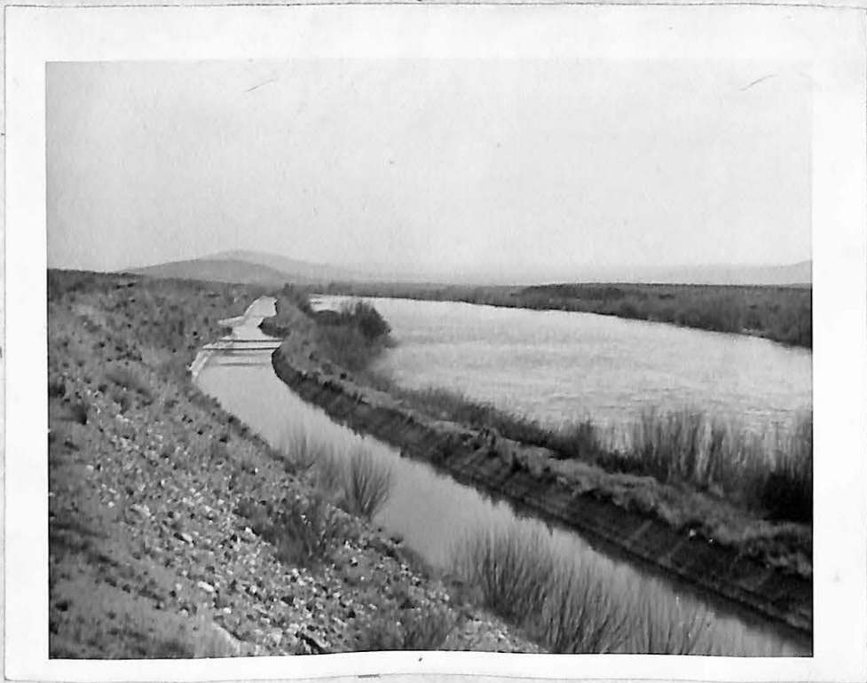
20. Main ditch supplying water to Richland area.
