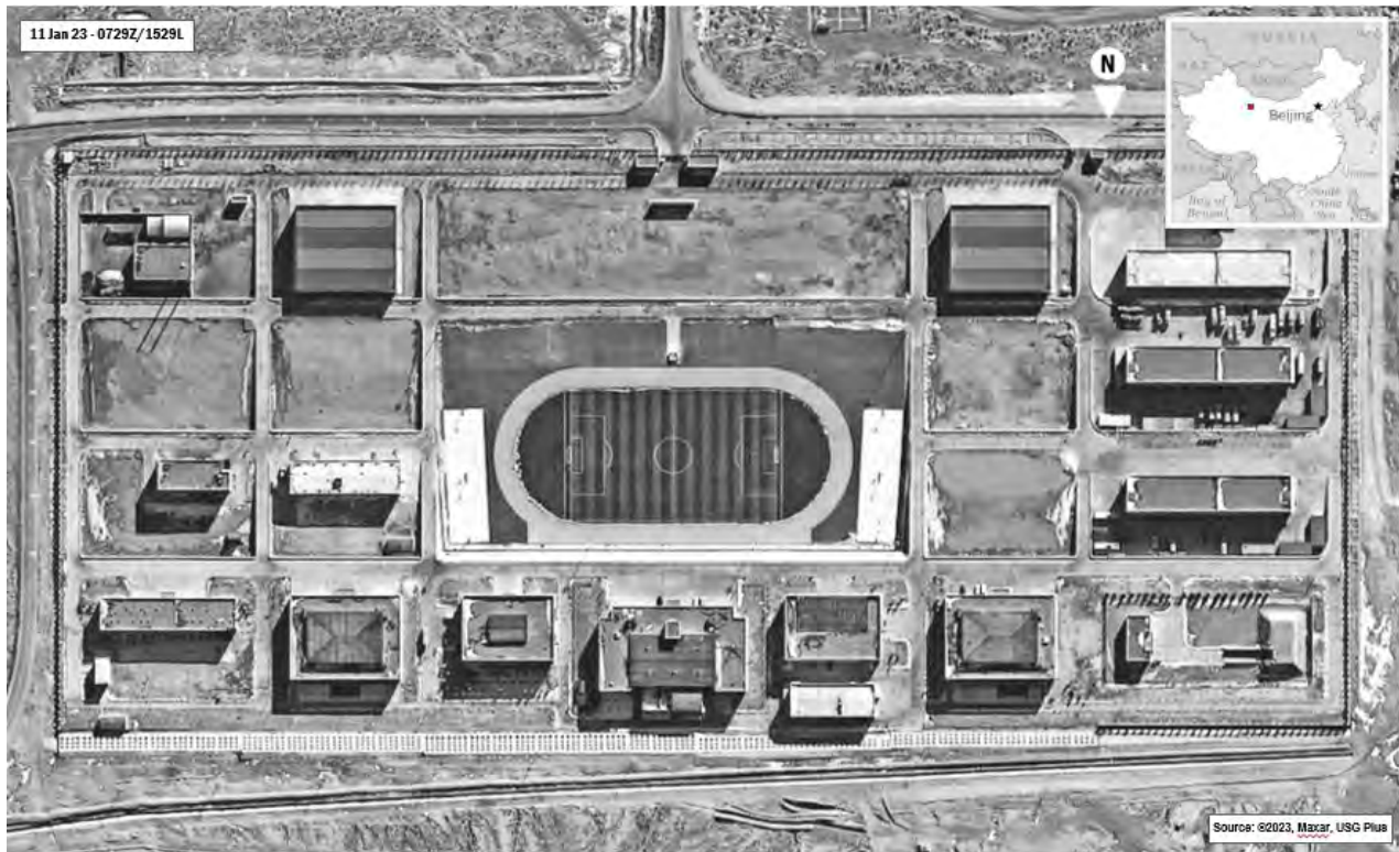
China: Military garrisons constructed at newly build ICBM Silo Fields – Guazhou ICBM Silo Field Missile Garrison
