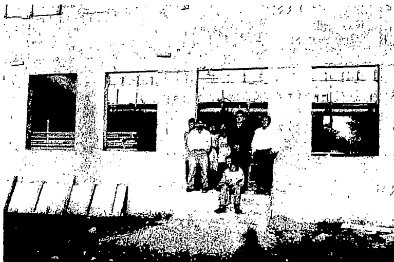
Community house under construction at Segakiato
